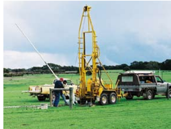
Piezometer construction (photo by Chris Henschke)
