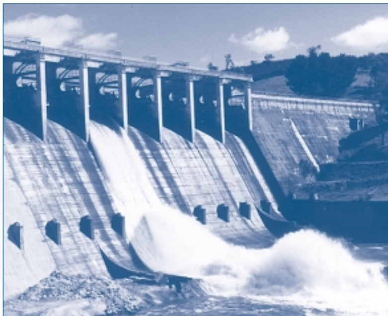
Lake Glenmaggie, located on the Macalister River in central Gippsland, is the water storage for the Macalister Irrigation District (MID), which is the largest of the three irrigation districts in southern Victoria. The lake holds some 191,000 ML, but the flow characteristics of the Macalister River can fill the lake twice over in a normal year. For this reason the Glenmaggie Weir is topped with fourteen radial gates, which can be opened to release water into the lower river at predetermined rates and thus avoid uncontrolled spills or floods threatening the downstream environment. In the picture, two gates are open to allow additional flows to pass. As well as this, essential environmental flow requirements are passed via the hydro electric power station located below the weir. Water can also be passed either directly into the river through an outlet tunnel or, in cases of extreme danger, into the MID itself via the main channel outlets.
