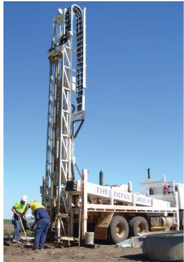
Figure 4. Typical drill rig for installation of an irrigation bore.
