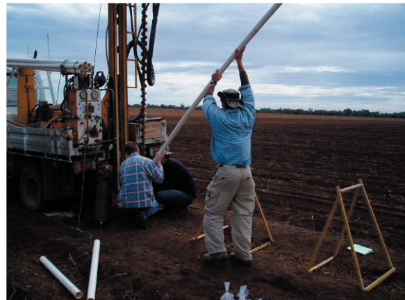
Chris Vanags hoists a piezometer into the air, in the final stages of installation in a cotton paddock in Moree.
