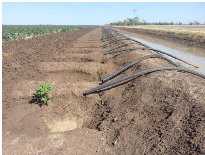
Figure 7. Traditional flood irrigation infrastructure
