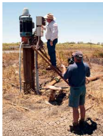
Greg Bath, DEEDI films Pat Daly of Daley Water Services who is inspecting a flood-inundated electric turbine pump to illustrate what growers need to do to repair pumps damaged by floods.
