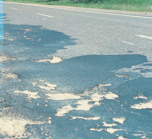
Road damage: a high cost reality for salinity
