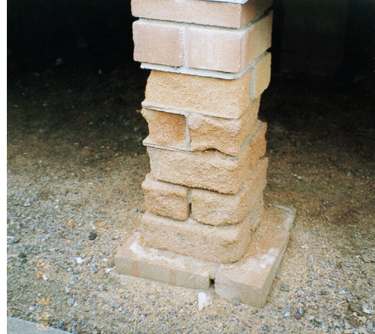
Salt attacking house foundations
