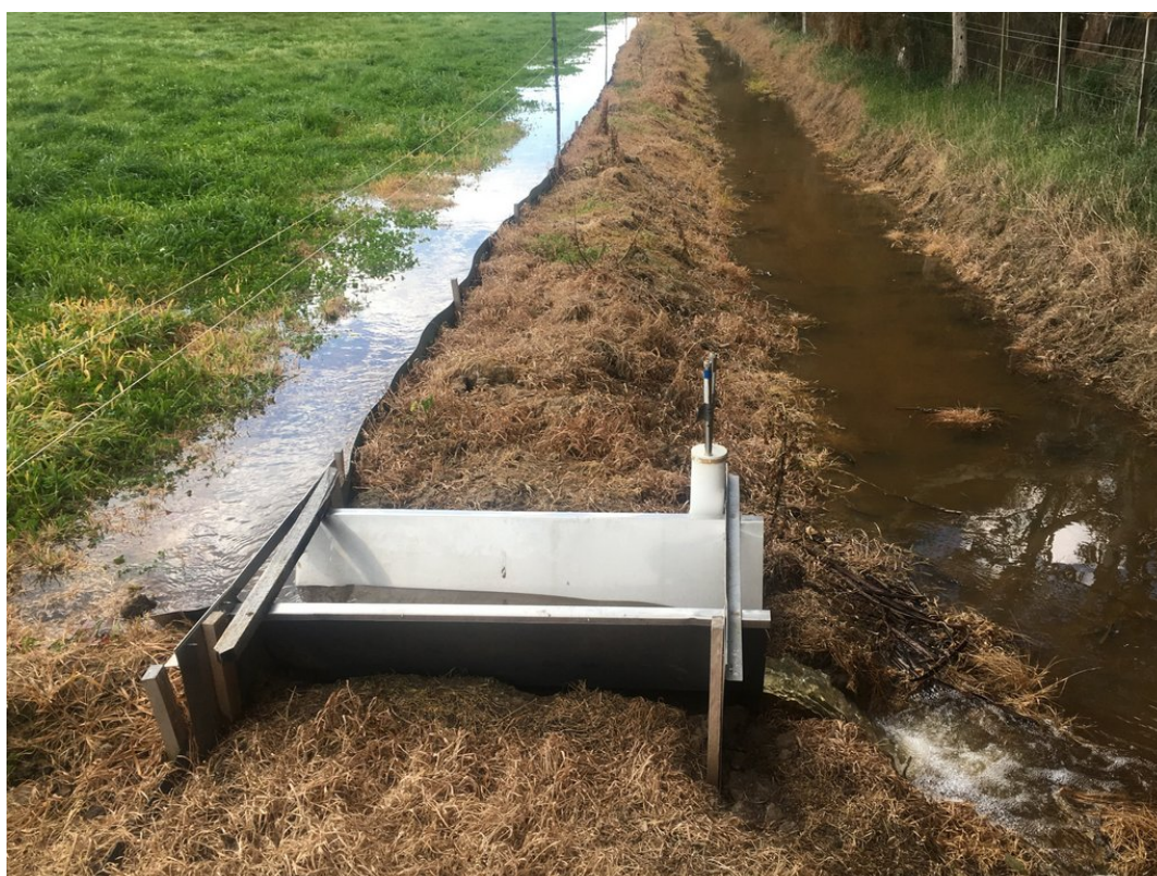
Figure 5: Bay runoff flume
