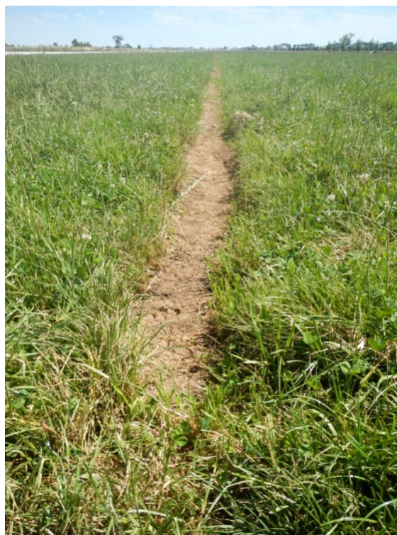
Figure 1: Shallow surface drain installed on a pasture bay
