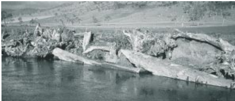
Logs and stumps used to rehabilitate banks.
