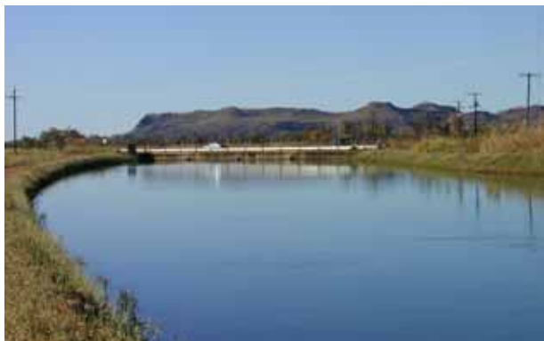
> The M1 irrigation supply channel in the ORIA.
