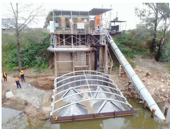
Figure 20: Installation of cone screens. Reproduced with permission from AWMA. https://www.awmawatercontrol.com.au/project/trangie-nevertire-irrigation-scheme-fish-screens
