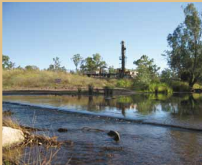
FIGURE 4: Establishment of deep piezometers.
