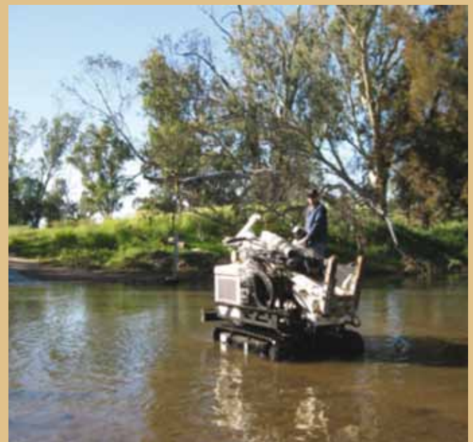
FIGURE 5: Installation of shallow piezometers.
