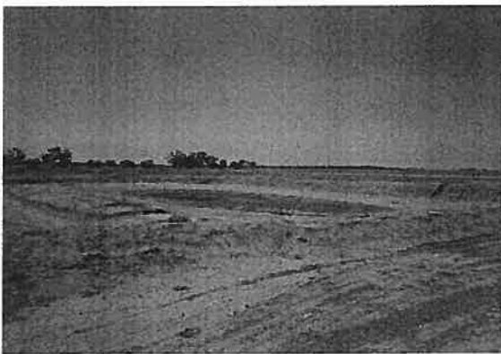
Photo 29: Unfenced, unlined evaporation pit
