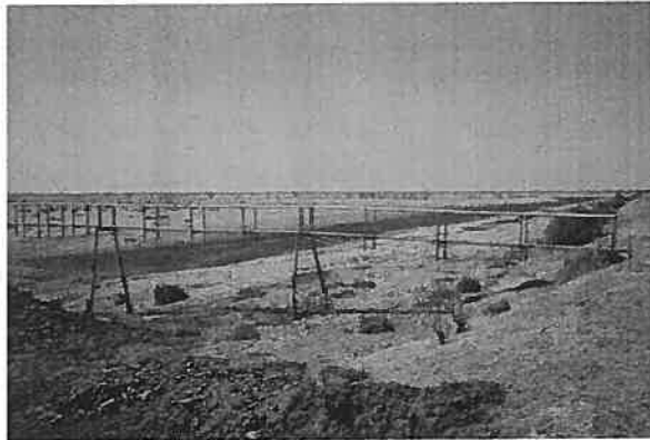
Photo 3: Typical large surface area water storage
