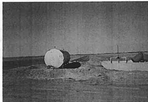
Photo 17: Earthen bunding around diesel tank adjacent to water distribution channel meets Australian Standards
