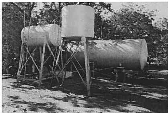
Photo 19: Lack of bunding or other protection measures around diesel and petrol tanks
