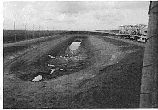
Photo 28: Fenced, unlined evaporation pit
