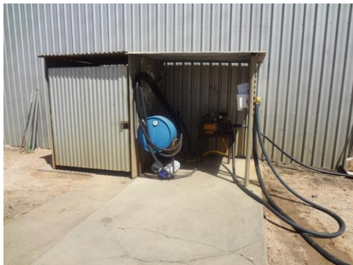
Wash down pad
