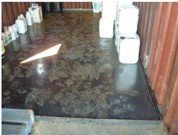
Floor in chemical shed (an old shipping container) is improved with the installation of metal bunding constructed on the farm.
