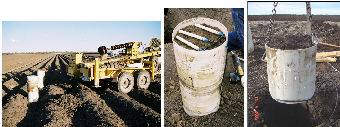
Figure 2. Installation of a lysimeter. (a) The “Proline” soil sampling rig, used to remove intact columns of soil, (b) the base of the lysimeter with the three ceramic candles in place and plumbed through the lysimeter wall, (c) the lysimeter after the base is sealed with a plastic disc (visible is the DD water collection tube) being lowered back down the hole.
