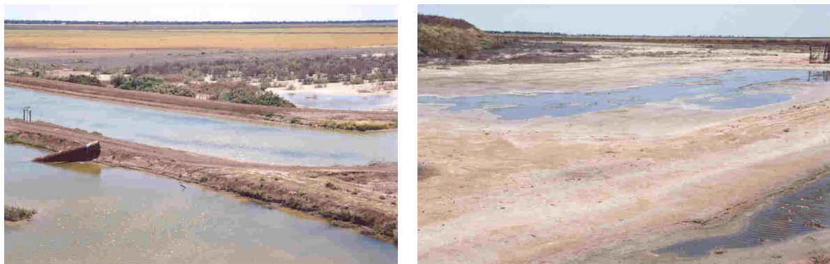
Figure 1. Water logging and soil salinisation adjacent to a) supply channel and b) water storage in the Bourke Irrigation District, Darling River valley.
