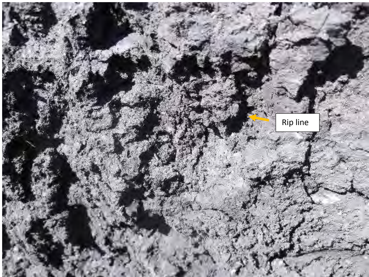
Ripped soil pit
