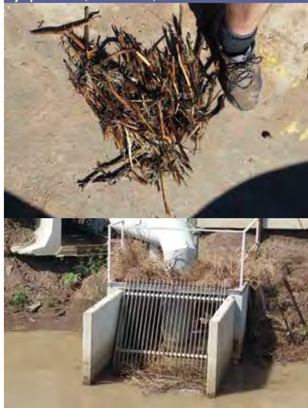
FIGURE 2: Cotton trash can reduce pump performance by up to 30%. (Photo: Phil Szabo)
