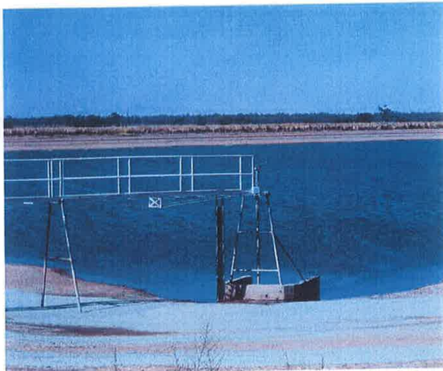
Figure 4. Federation Farm dam inlet
