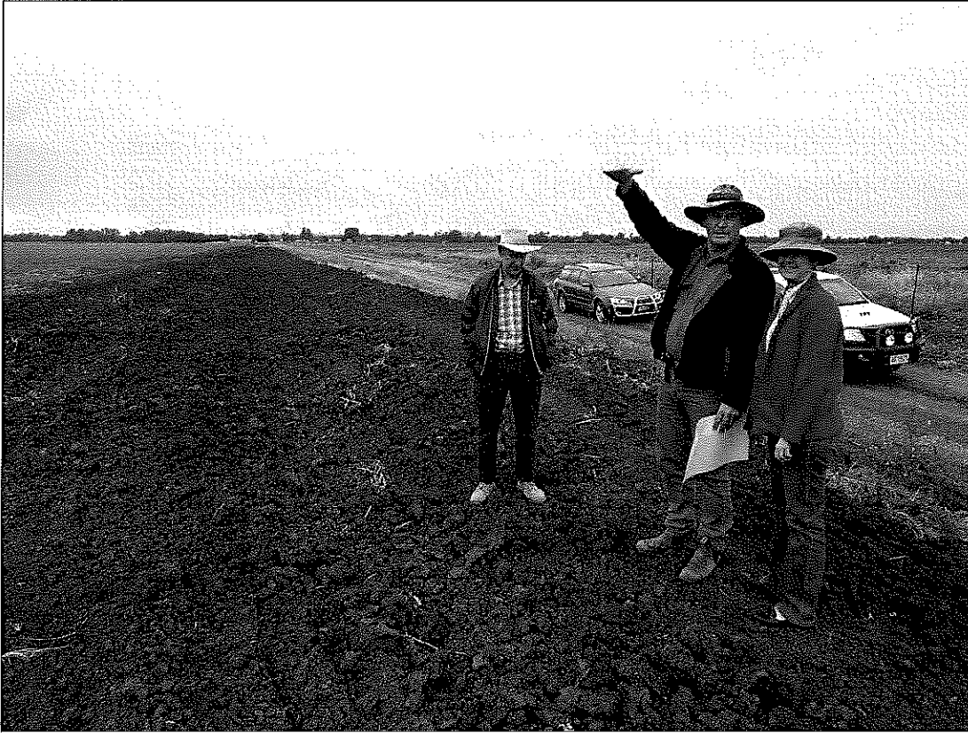
Fig7 : During a site inspection of proposed repair works Dawn and Peter French (Theodore) reflect on the height of the 2010/11 devastating flood across their cotton fields and the severe infrastructure damage they caused.
