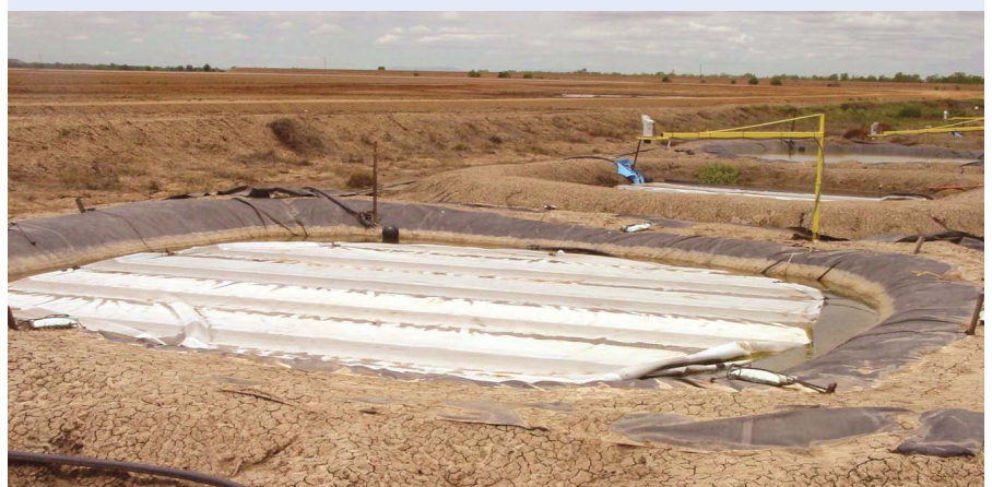
Figure 1.6.18 Covered and lined dam. Polypropylene liner and polyethylene cover
