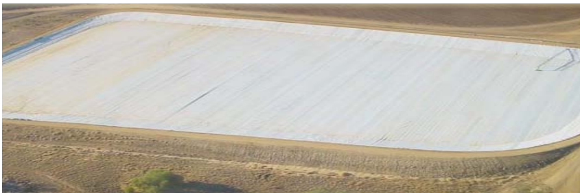
Figure 1.6.13 – A floating cover installed on a 4 hectare dam near St George, Qld.
